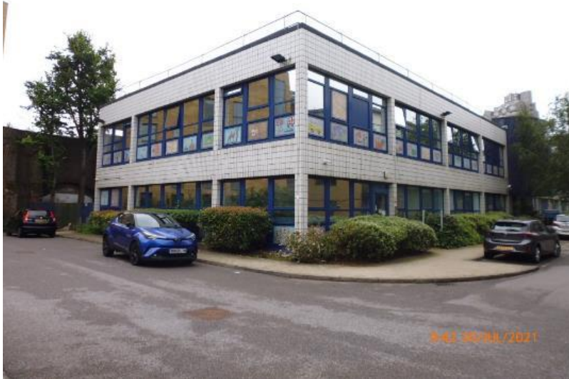
Figure 6 - Wooden Spoon House, Dugard Way.
