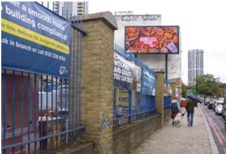
Figure 3 – The frontage to Kennington Lane is particularly unpleasant for pedestrians and dominated by a large, discordant billboard on the site.
