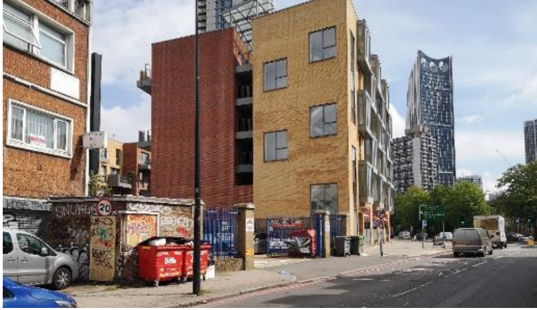
Figure 4 - The eastern end of the site frontage to Kennington Lane showing neighbouring property and the cramped and cluttered frontage treatment of the site.
