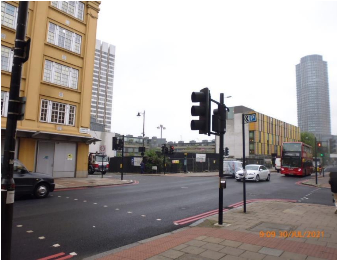
Figure 4 - Looking west from corner of Coin St and Stamford St towards the site.
