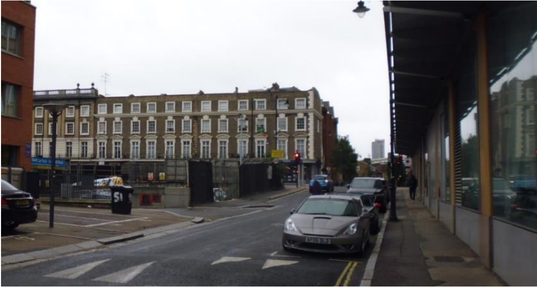
Figure 8 - Seen from Cornwall Road, the car park access ramp is on the left.
