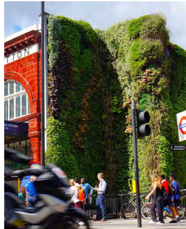
Living Wall (Edgware Station, London)
