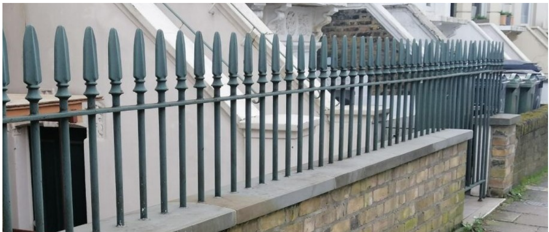
Figure 24 The railings at no. 25 provide a template for future reinstatements.
