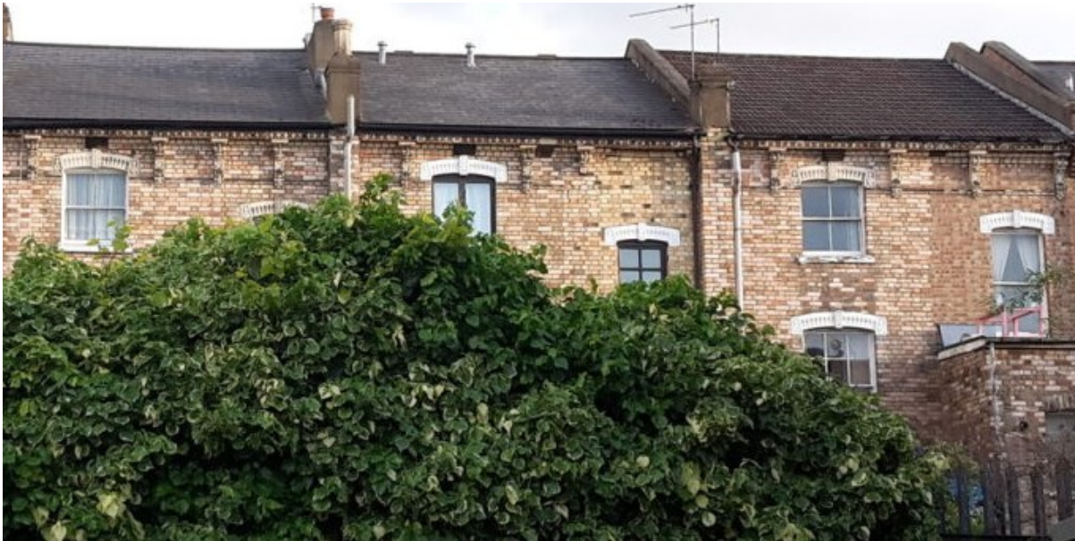
Figure 21 Some properties have gault brick rear elevations and fancy terracotta detailing
