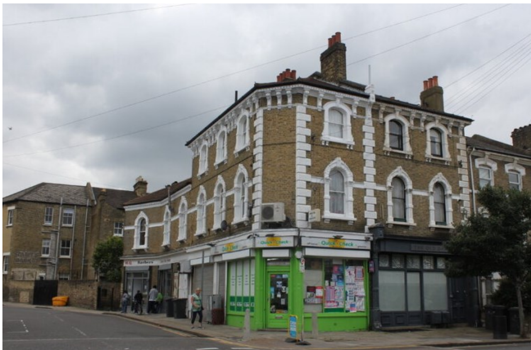
Figures 27 Statutory listed buildings on corner of Ferndale Road and Tintern Street.
