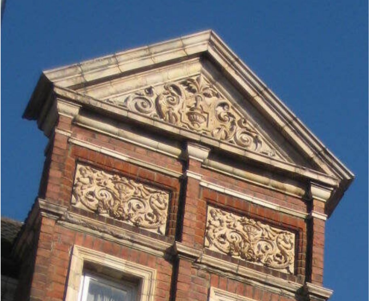
Figure 9 The gable panel of Rathcoole House's Ferndale Road elevation.
