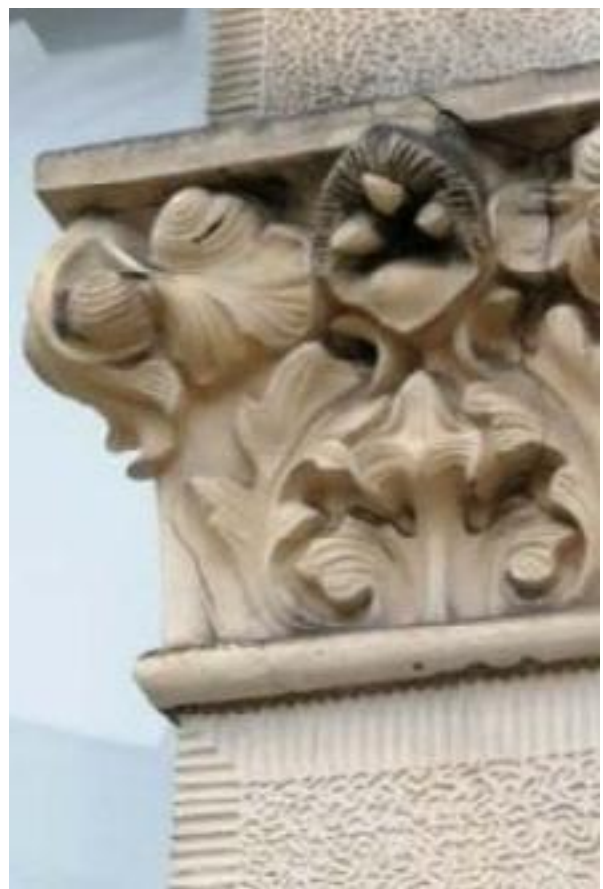
Figures 17,18 and 19 The precision of the terracotta moulding is impressive
