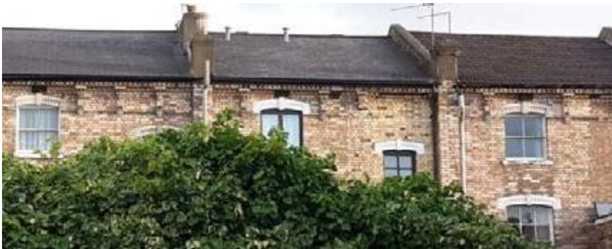
Figure 21 Some properties have gault brick rear elevations and fancy terracotta detailing
