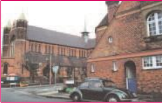
Matching materials: St. Margaret's church. In foreground matching orange brick tile-hung gable. Note coarse-rendered niche.
