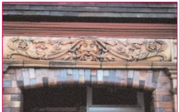
Terracotta door canopy detail.
