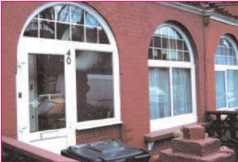
PVCu porch enclosure and inauthentic PVCu windows.
