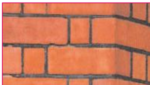
Good original pointing
