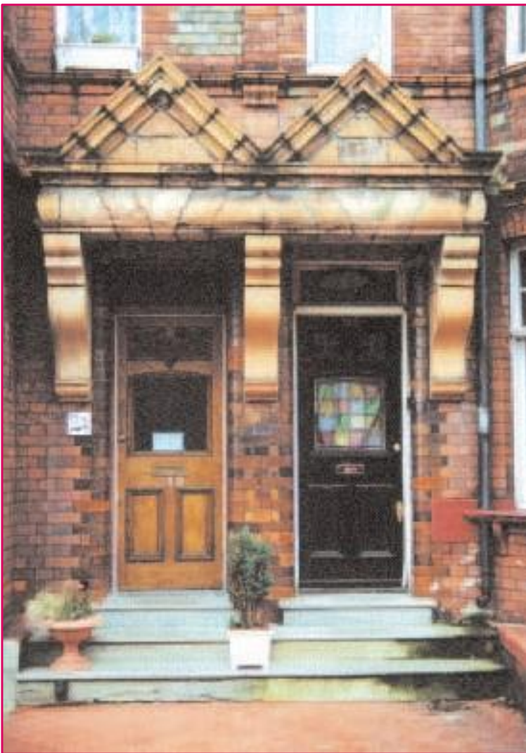
A pair of doorways with terracotta canopies and coloured glass. Note the diamond tiled forecourt.
