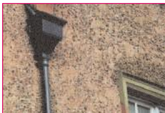
Original cast iron hopper and downpipe
