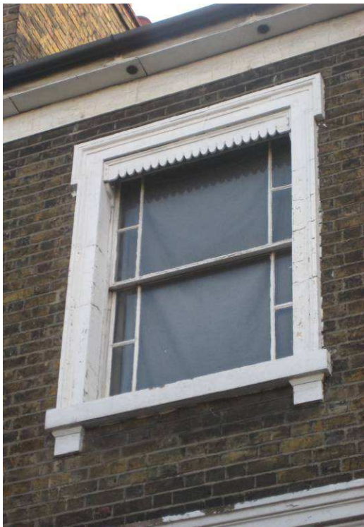
Finely detailed timber sash window.
