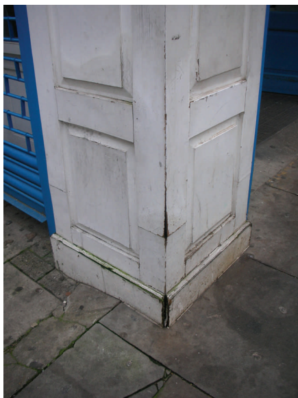
MDF stallrisers rot with the damp.
