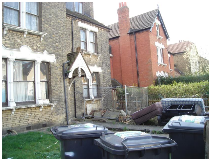
Photo 4: Dumping and poorly maintained external area
