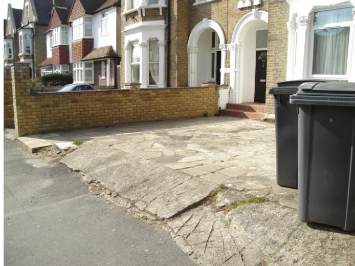
Photo 2: Poorly defined and maintained boundary
