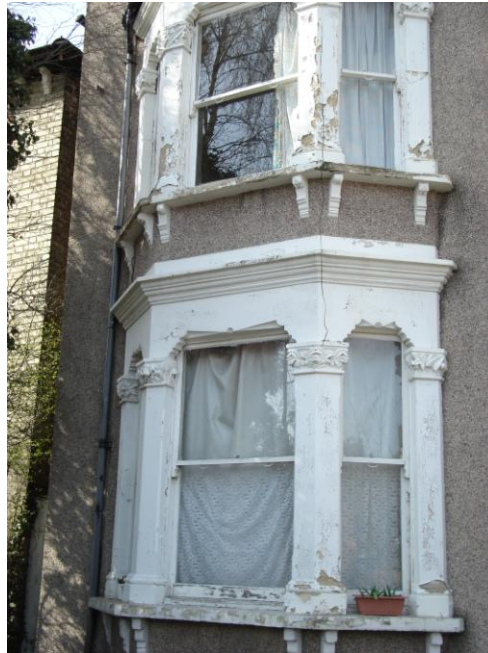
Photo 1: Poorly Maintained Facade
