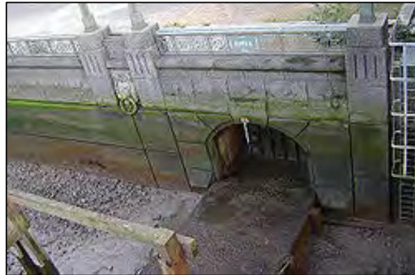
Figure 6.2: Effra Sewer outlet at Vauxhall Bridge
