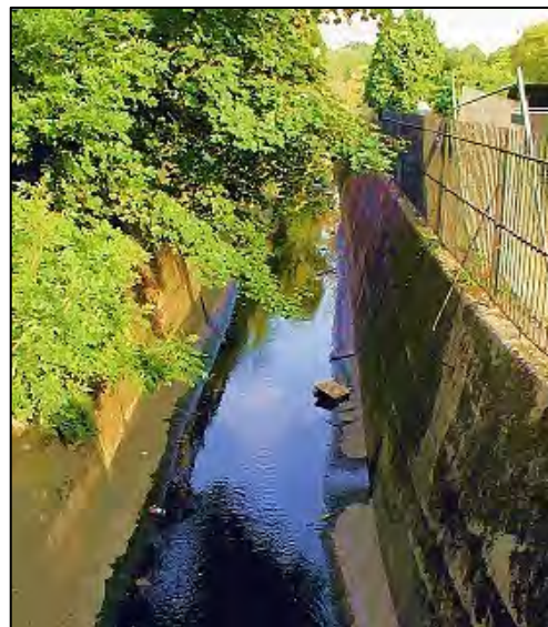
Figure 6.1: Typical section of the River Graveney
