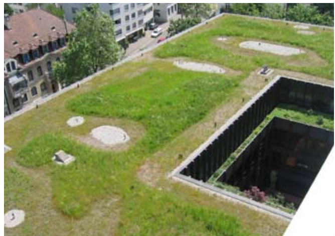
Green Roof on a large scale
