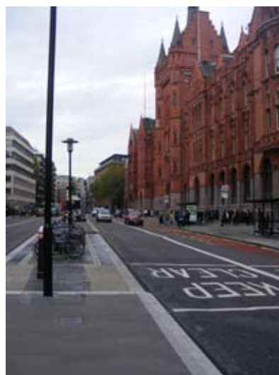
Road improvements on High Holborn
