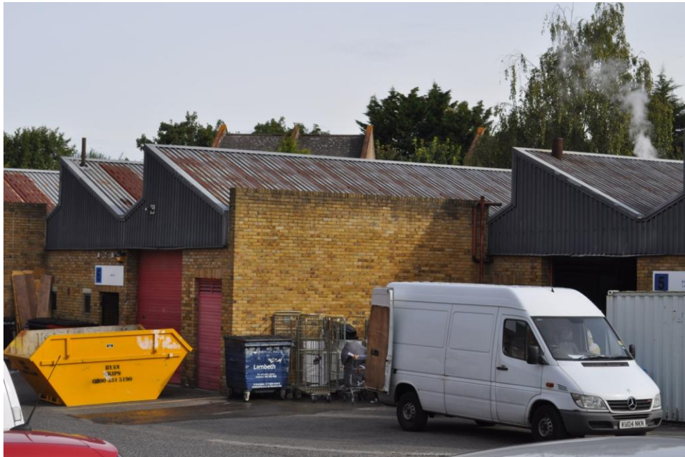
Figure 17. Hamilton Road Industrial Estate
