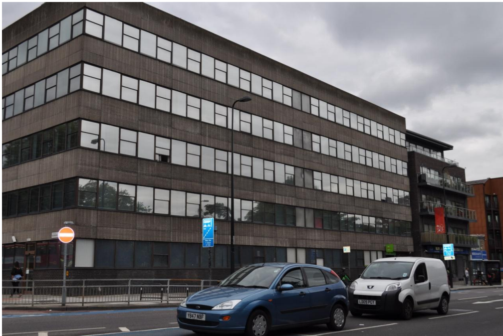
Figure 29. Office premises fronting onto Kennington Park Road
