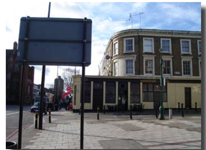
Irregular pavement widths and haphazard street furniture on Parade 1
