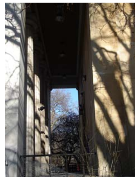
St Mark's Church: overgrown undergrowth
