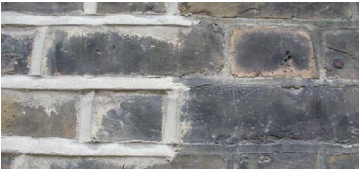
Modern 'weather-struck' pointing in modern cement (left) causes harm to brickwork.
