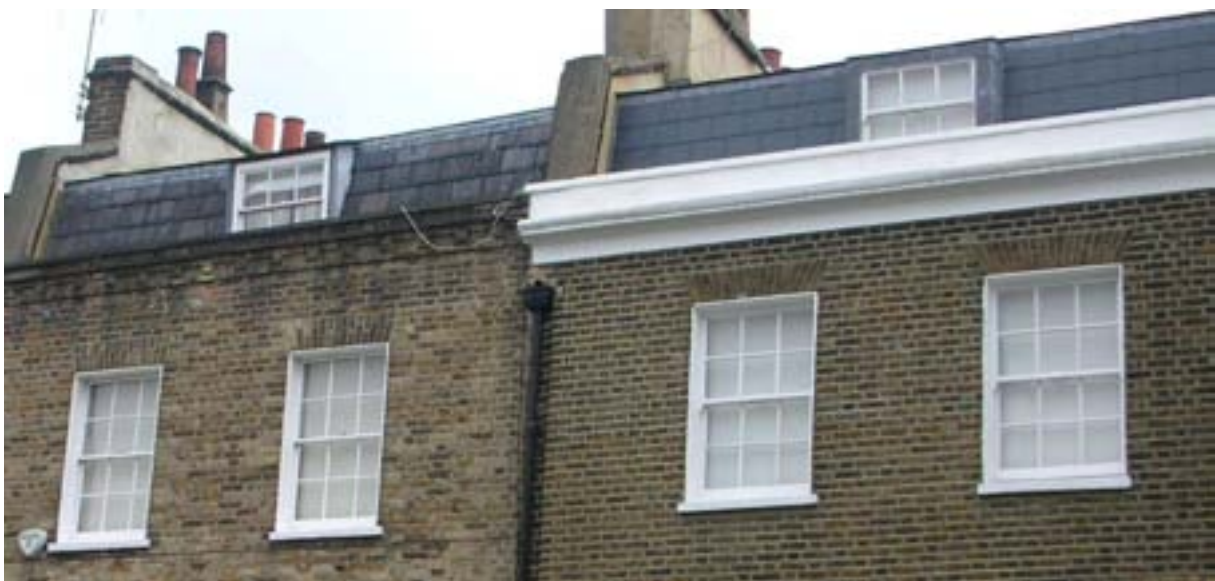
The stucco cornice on the right is authentic whilst the brick one on the left is a poor repair.
