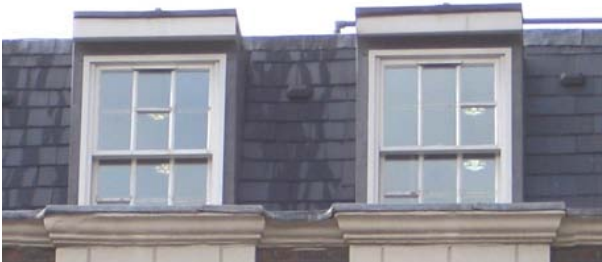
These stick-on glazing bars have dropped leaving an unacceptable appearance.
