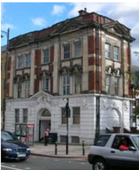
A) former Clapham Public Hall
