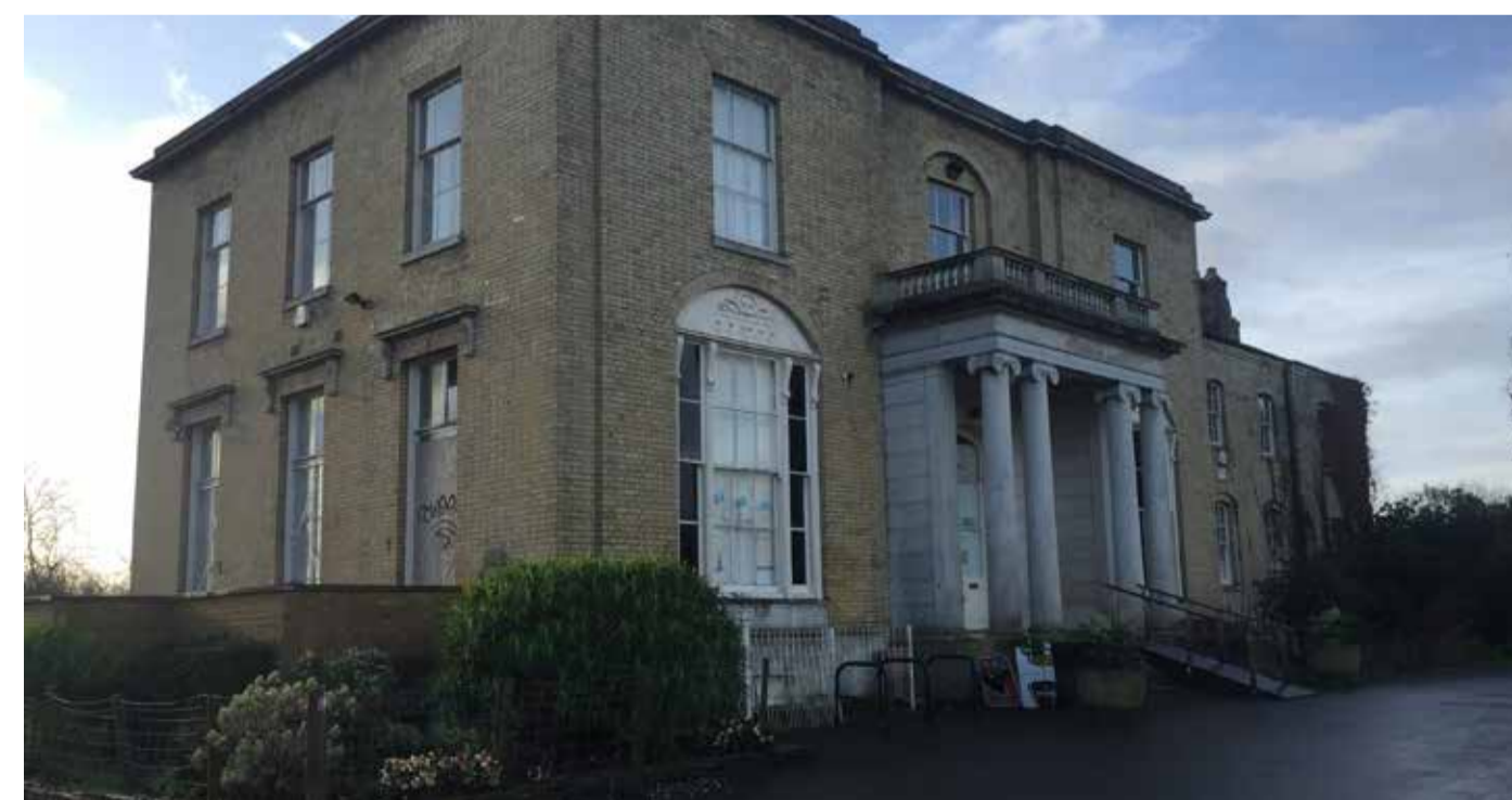
Neglect of the Hall has resulted in boarded up windows and graffiti.
