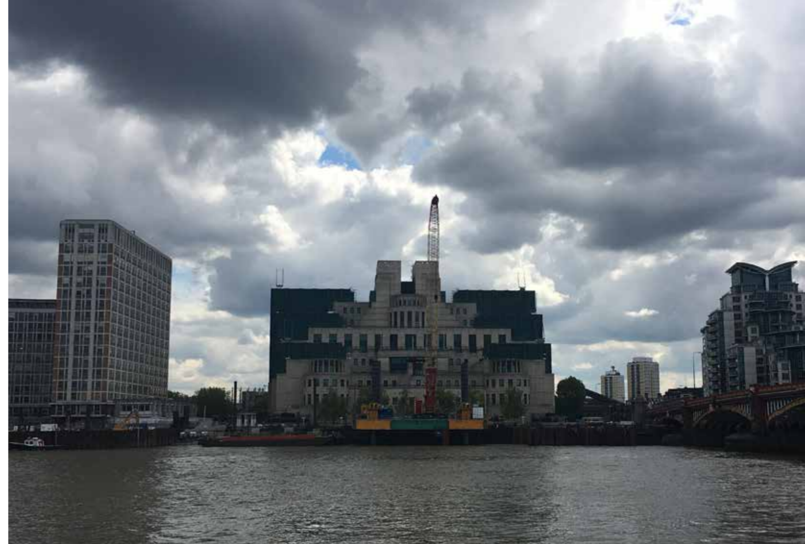
View: Terry Farrell's landmark MI6 building - April 2019
