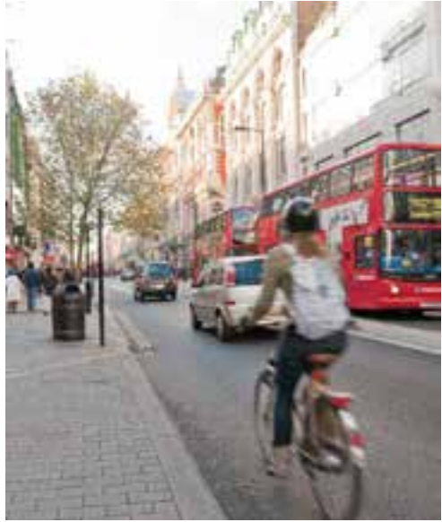
Oxford Street East where the redevelopment maximises the useable space and includes an innovative street layout called 'smooth stops'. This approach removes the need for bus laybys, so retaining space for pedestrians and smoothing traffic flow. This is reinforced by a median strip to provide safe, informal crossings, a consistent kerb line and a dedicated street furniture zone.
