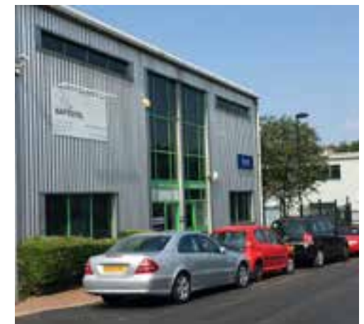
Industrial development, Windsor Grove, West Norwood
