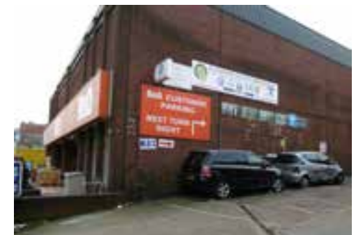
Access to B&Q's car park
