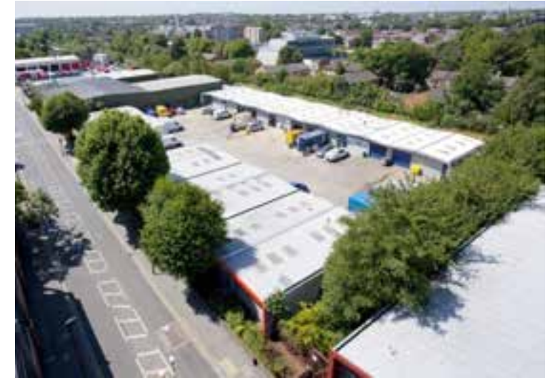
Flexible small industrial units in Herne Hill
