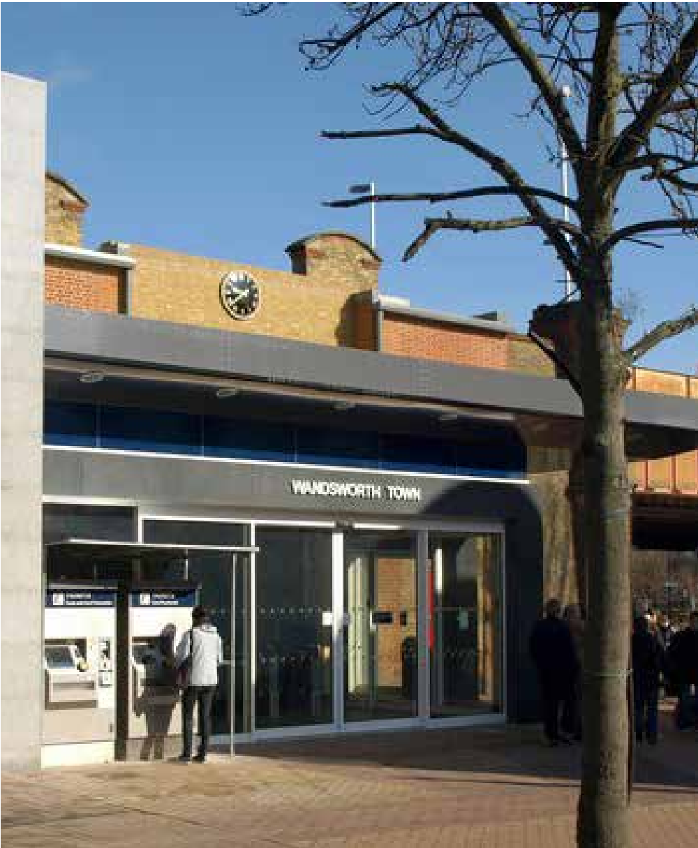
Wandsworth Town station improvements
