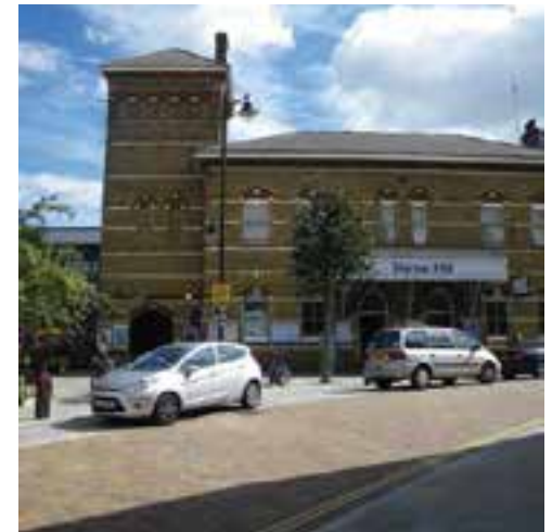
Tulse Hill station scheme where a major part of the design involved closing the station on Railton Road to through-traffic. A raised table outside the station and shared surfaces made of Yorkstone have provided a high-quality pedestrianised environment.
