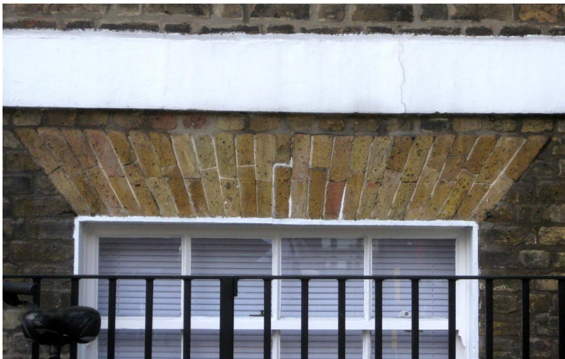
Poorly executed brick repairs can cause significant harm to buildings.
