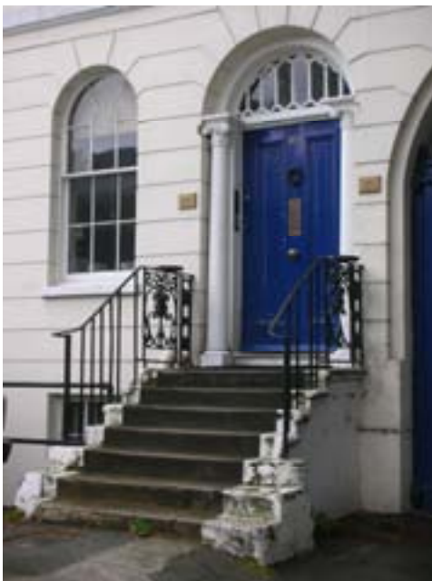
Carefully detailed ironwork or walls typically retain front entrance steps.
