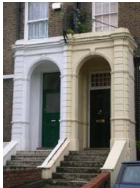
Carefully detailed ironwork or walls typically retain front entrance steps.
