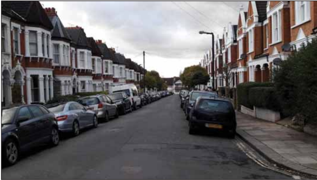
Figure 45. Norfolk House Road
