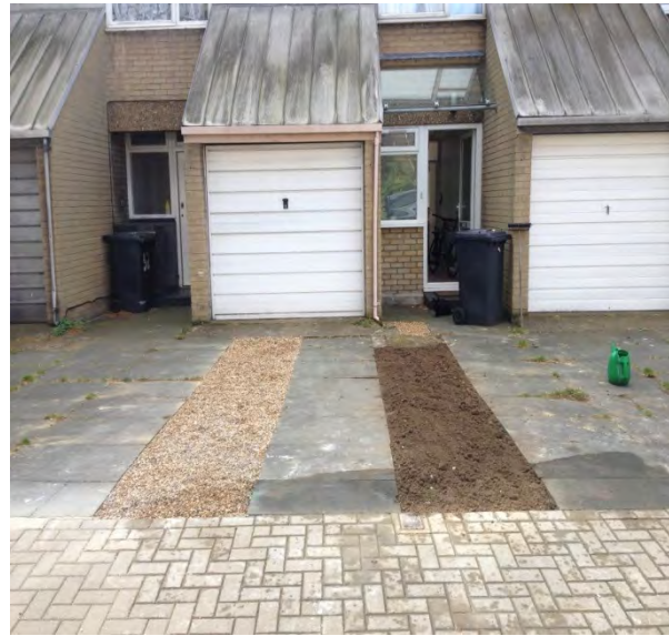
Reedworth Street after Depave Retrofit
